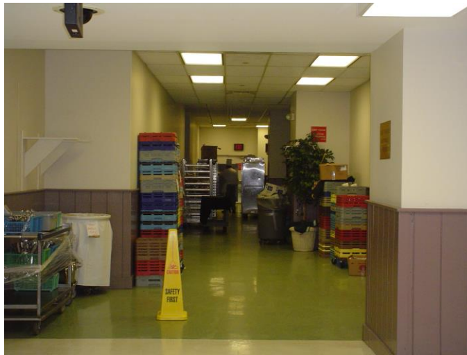
This is an obstructed means of egress.
