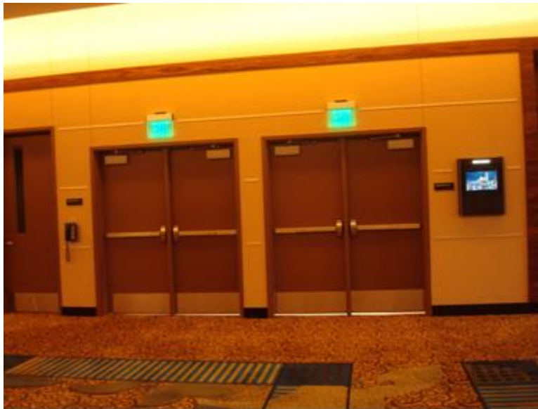
Exit: an exit is that portion of a means of egress that is separated from all other parts of a building or structure by construction or equipment as required to provide a protected way of travel to the exit discharge, such as stairways.
